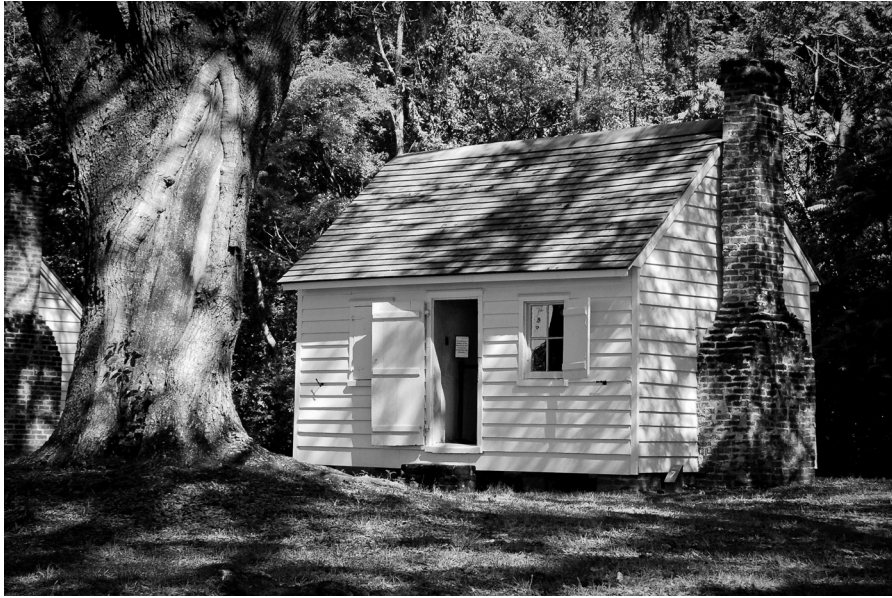
In 1990, John Gathers, a descendent of Hanna and Gable Gathers, both enslaved by the McLeod family, was living in this former slave dwelling. (Photo courtesy of the Charleston County Park and Recreation Commission)
