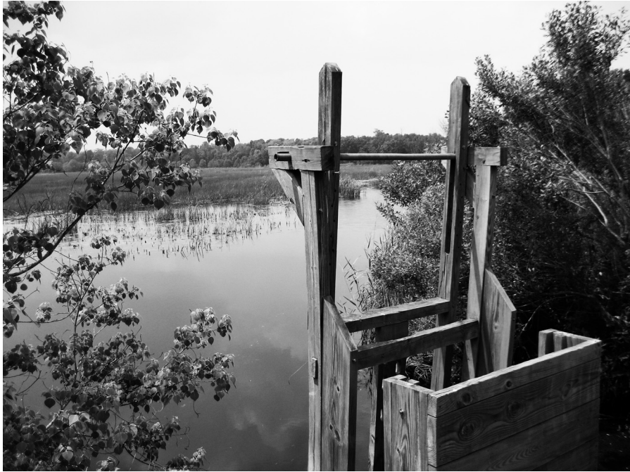
Rice trunk used for irrigating former rice fields at Caw Caw, ca. 2000. (Photo courtesy of the Charleston County Park and Recreation Commission)
